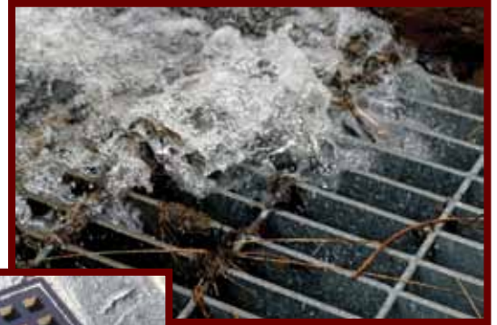
Stormwater enters the storm drain through this catch basin grate.
