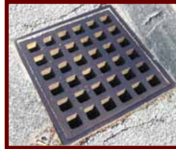
Stormwater enters the storm drain through this catch basin grate.
