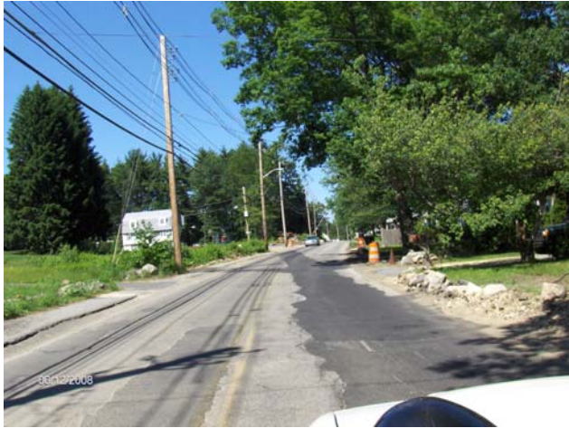
Drainage installation - Cook St
