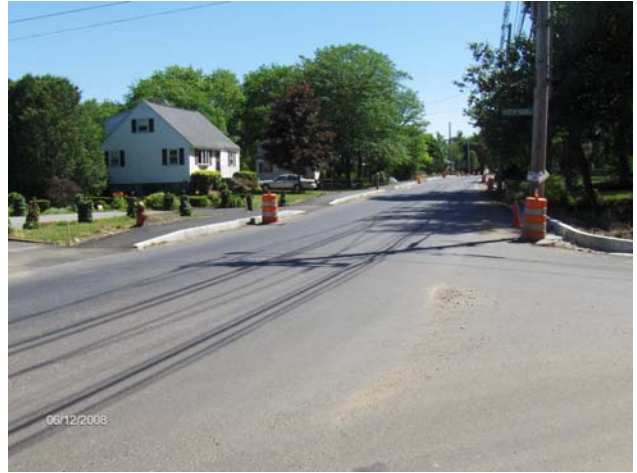
New curb/sidewalks/pavement - Cook St
