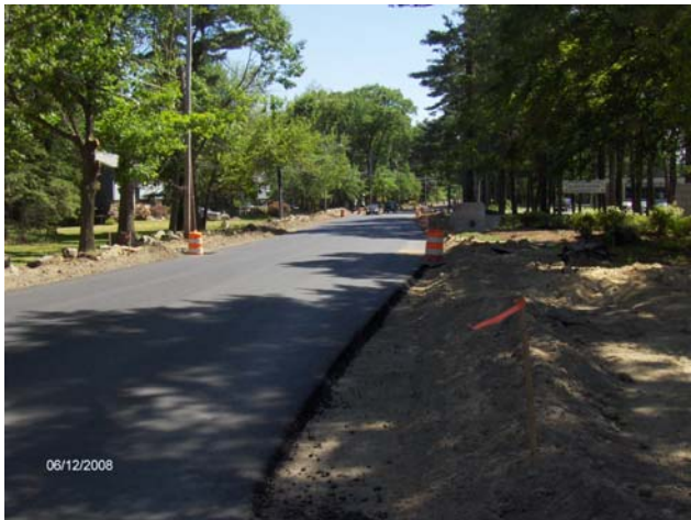
Base course pavement - Cook St
