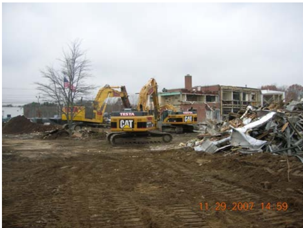
Filter Building Demolition
