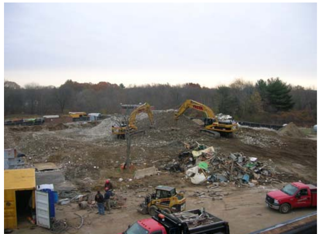
Pretreatment Building Demolition
