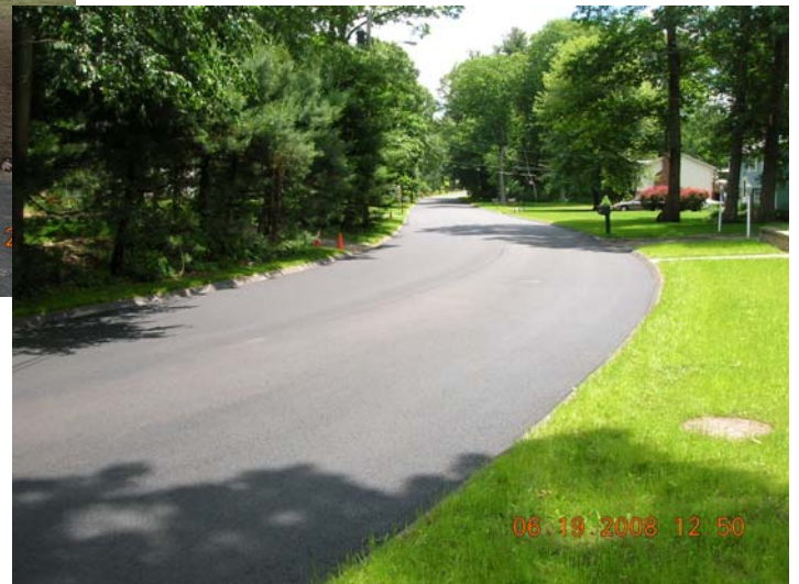
Final Paving - Theresa Avenue
