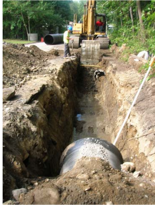
Drainage installation on Michael Rd
