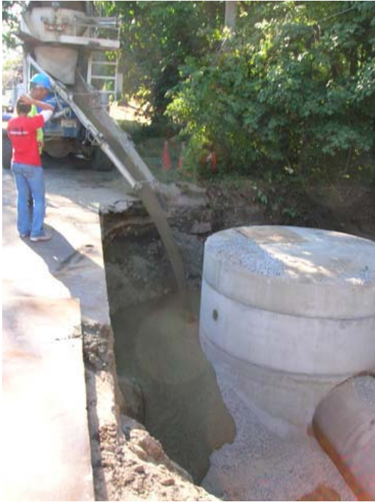
Drainage installation on Sheldon St
