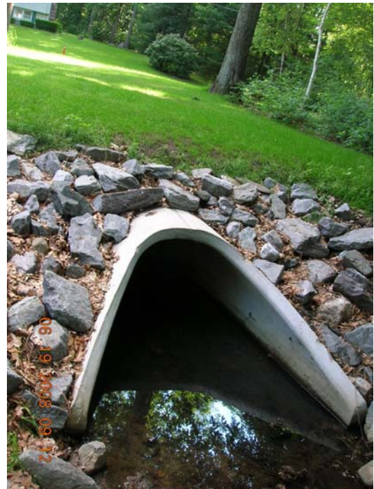
Drainage pipe at Theresa Avenue
