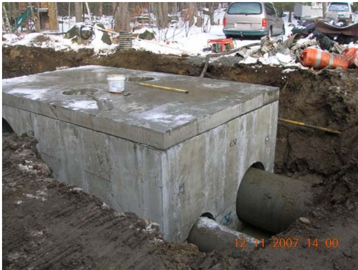
Drainage manhole installed for stormwater storage on Michael Road
