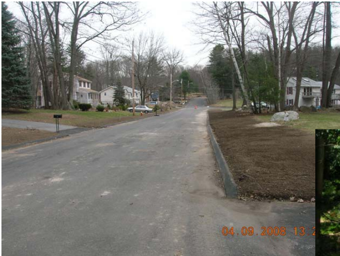
Loam placement on Crooked Spring Rd April 2008 before final paving
