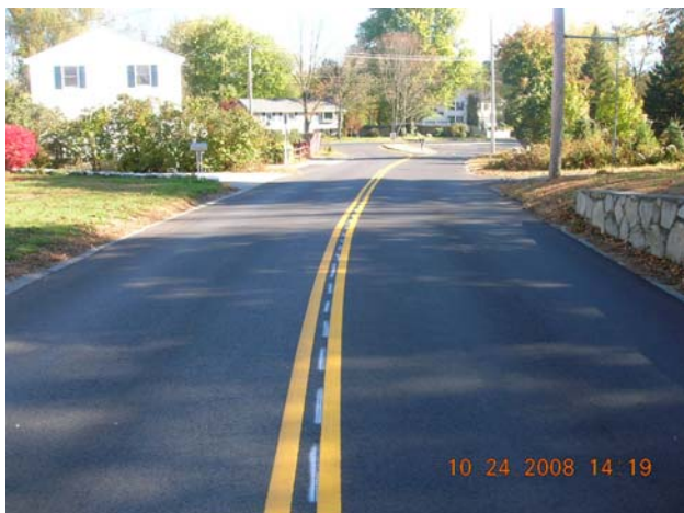
Allen Road Extension – Completed
