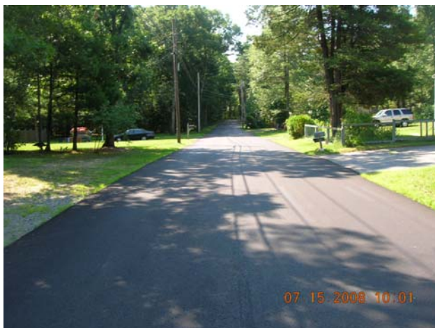
Connolly Road Final Paving
