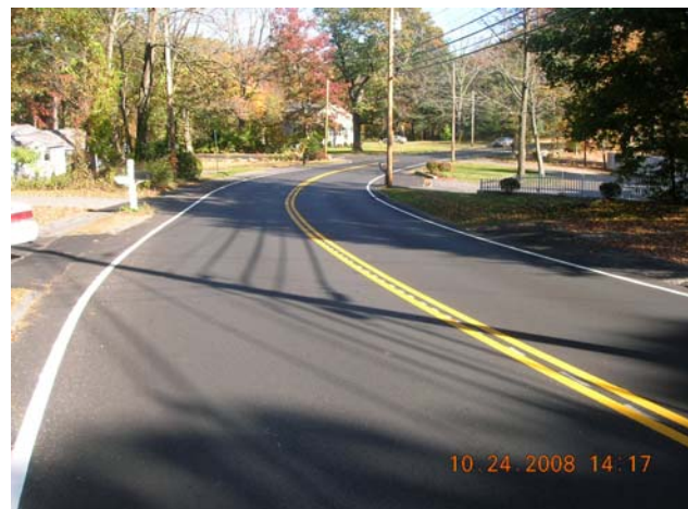
Andover Road – Completed
