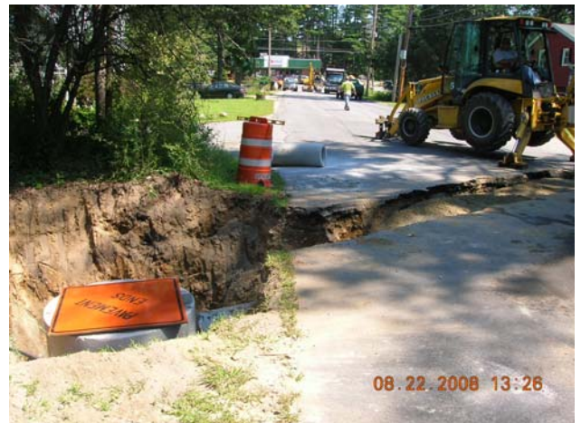
River Street –Aug 2008 Drainage Installation
