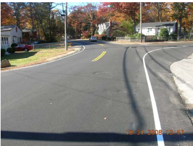
River Street Final Paving – Oct 2008
