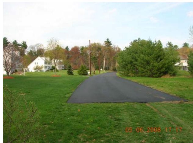
Forest Street Final Paving
