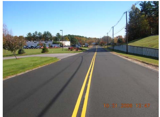
Esquire Road – Final Paving– Oct 2008
