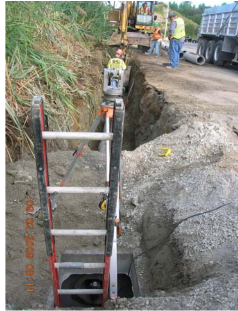
Republic Road – Drainage Installation
