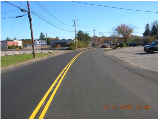
Republic Road – Final Paving– Oct 2008
