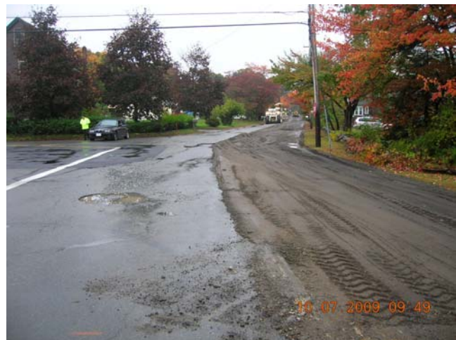
Roadway Reclamation – High Street
