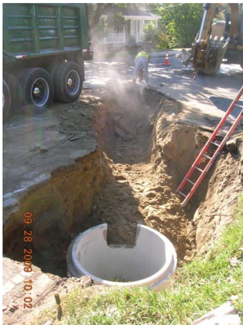
Drainage installation – High Street
