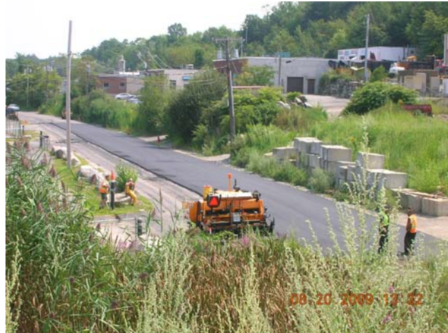
Republic Road Paving
