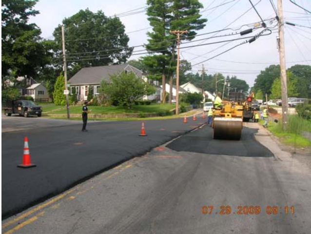
Bridge Street Paving
