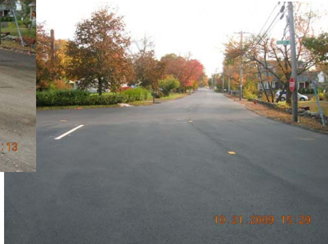
Final Paving – High St @ Sheldon St
