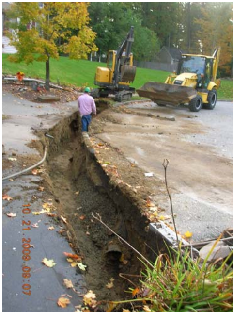
Subdrain installation – Margaret Lane
