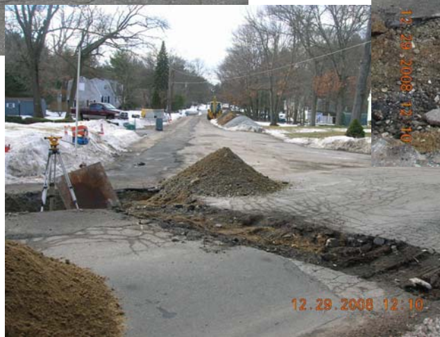
Drainage installation – Oak Street
