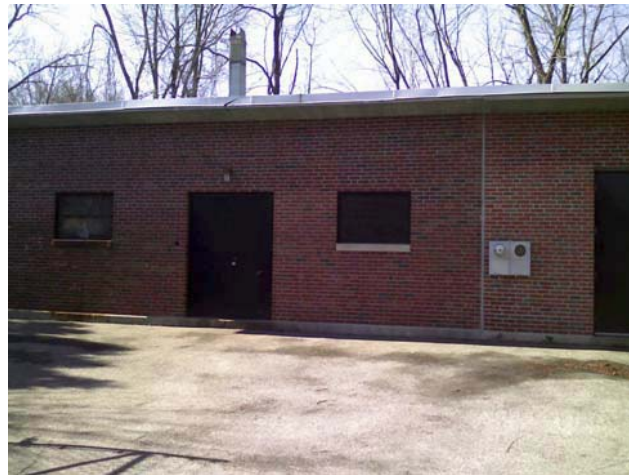
Rogers Street Pump Station
