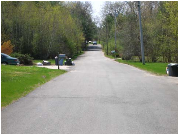
Greenleaf St after Sewer
