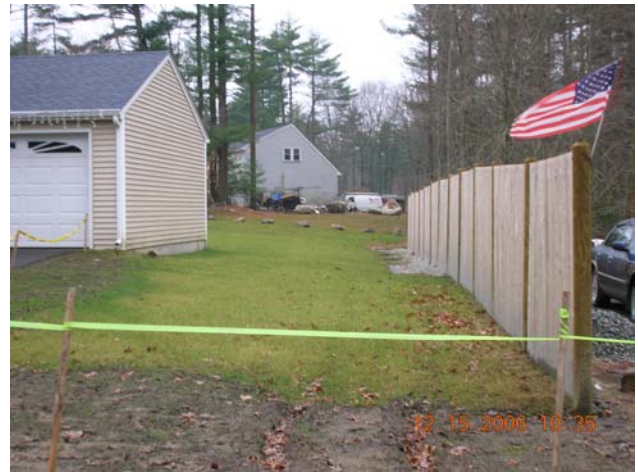
Connolly Rd Easement after Sewer
