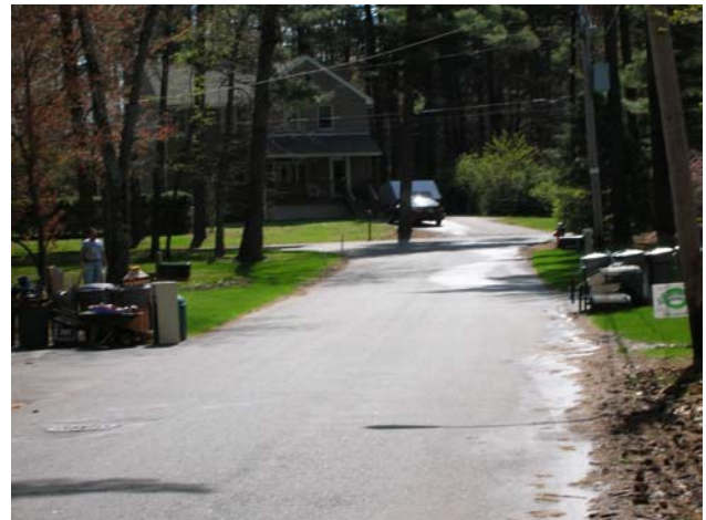
Green St after Sewer
