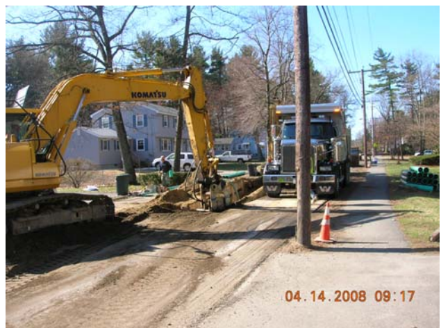
Baldwin Road Sewer Main installation – April 2008
