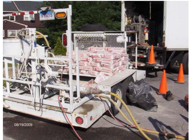
Equipment Trailer for Invert Sealing
