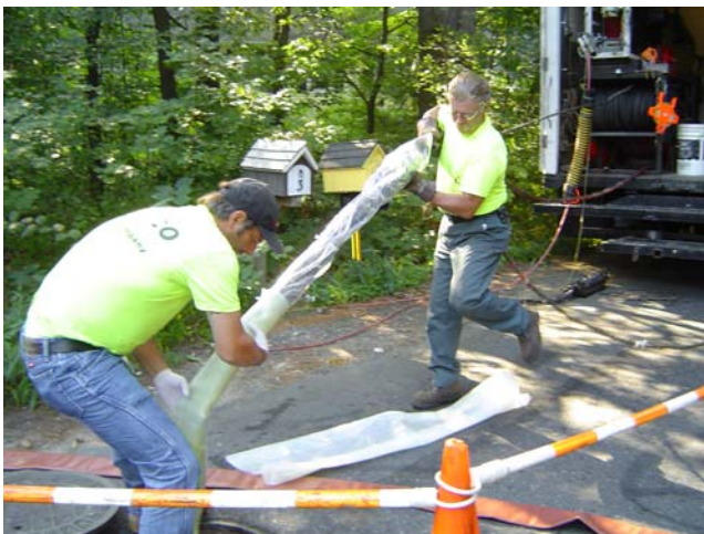
Placing short liner in pipe
