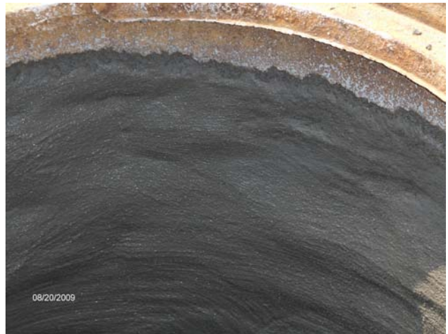
Newly sealed manhole chimney
