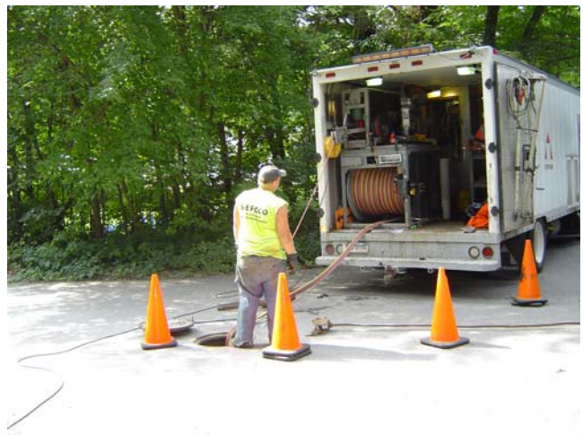
Contractor monitoring the inspection
