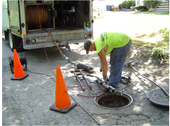
Packer and camera being prepared for 8" line
