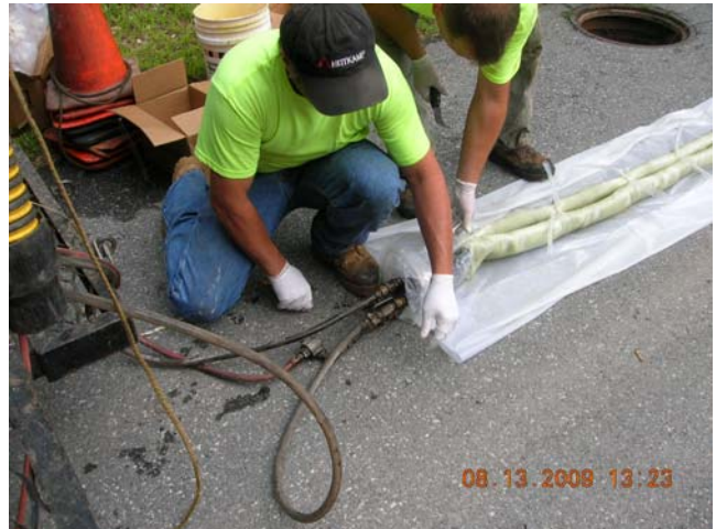
Short liner being prepared for installation
