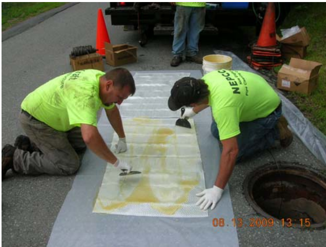
Short Liner being impregnated with epoxy resin
