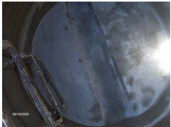
Newly cleaned, lined and sealed manhole
