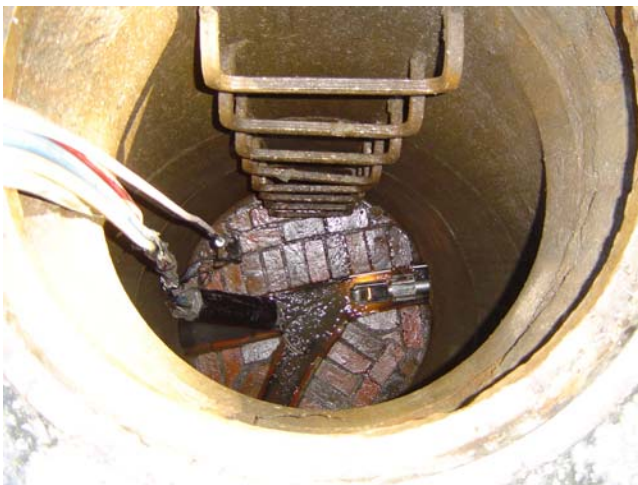
Packer and camera being installed
