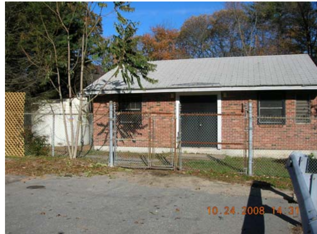
Pump Station – Exterior
