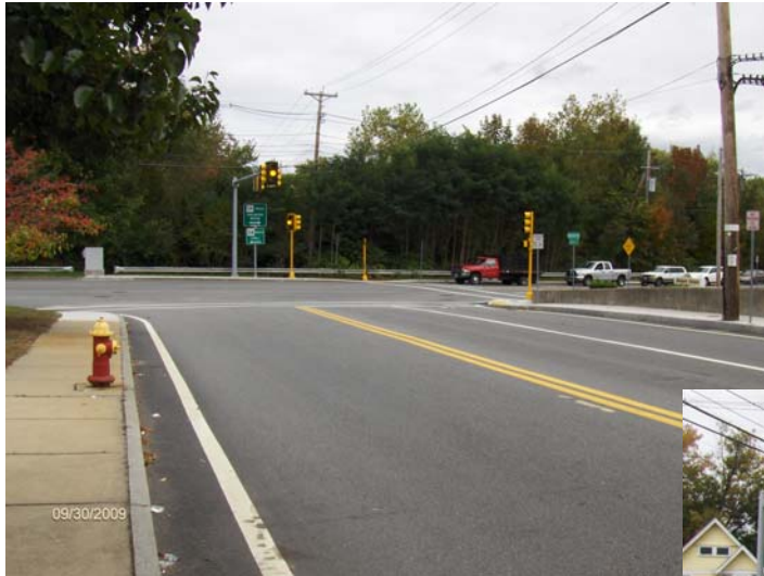
Boston Rd @ Bridge St
