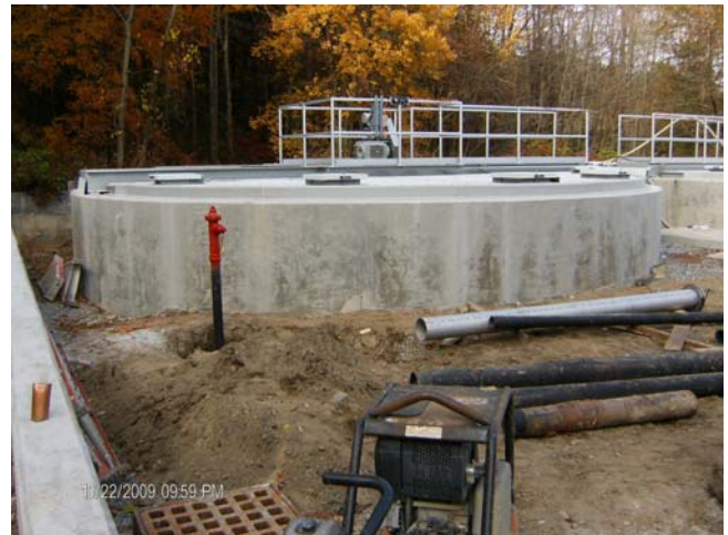
Gravity Thickener and Piping Installation
