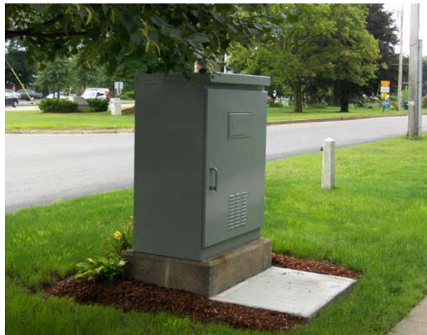
New Controller Installed on Old Foundation
