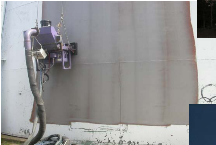
Robot removal of existing paint
