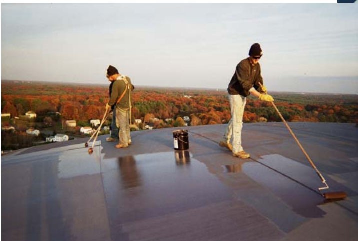
Working on the roof.
