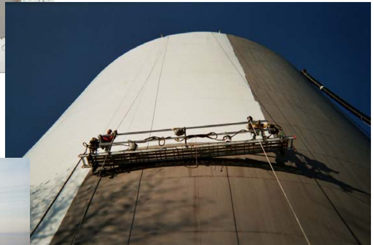
Final coat of paint being applied
